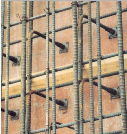
Instead of drilling, simply nail the Form Saver onto the form.
