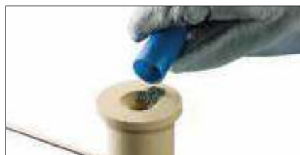
Fig. 14 Pour the starting material onto the Cadweld One Shot cover.
