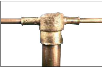
Fig. 17 You are ready to make another Cadweld One Shot connection.
