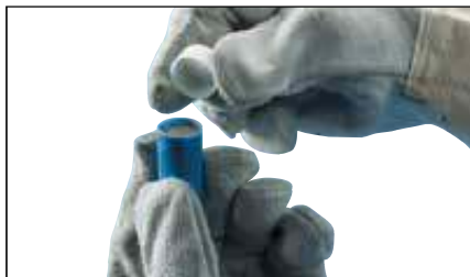
Fig. 10 Next, take the tube of welding material included in the Cadweld One Shot package and remove the lid over the crucible.
