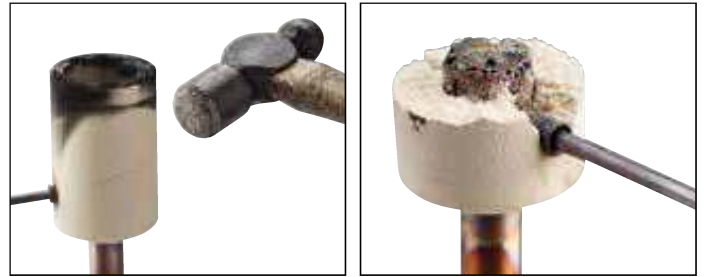
Fig. 15 Break the ceramic Cadweld One Shot mold off of the connection. Avoid contact with hot materials. See the "nVent ERICO Cadweld Quality Standards" section to see whether a quality connection has been made.
