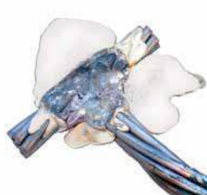
Reject. Fill too low. Weld cavity was not filled over cable strands. "Fins" indicate that the mold was not closed tightly due to incorrect mold, incorrectly adjusted handle clamp, or presence of foreign material in mold parting line. Before making the next connection, check the mold for each of the above.
