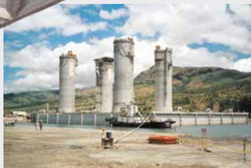
Malampaya Offshore Platform – The Philippines
