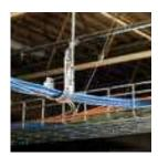
Material: Spring Steel Finish: nVent CADDY Armour
