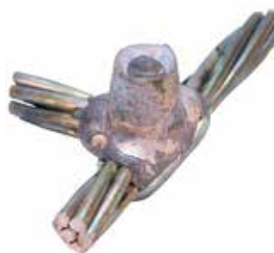
Reject. Extreme amounts of slag on surface are caused by welding material leaking past disk or complete lack of disk. Inspect the condition of mold disk seat and check disk positioning prior to making the next connection.
