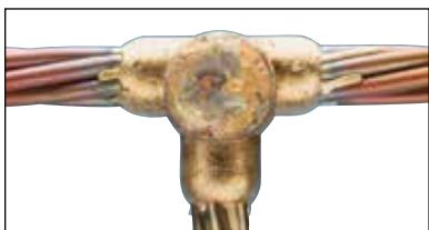
Fig. 23 Completed Cadweld connection.
