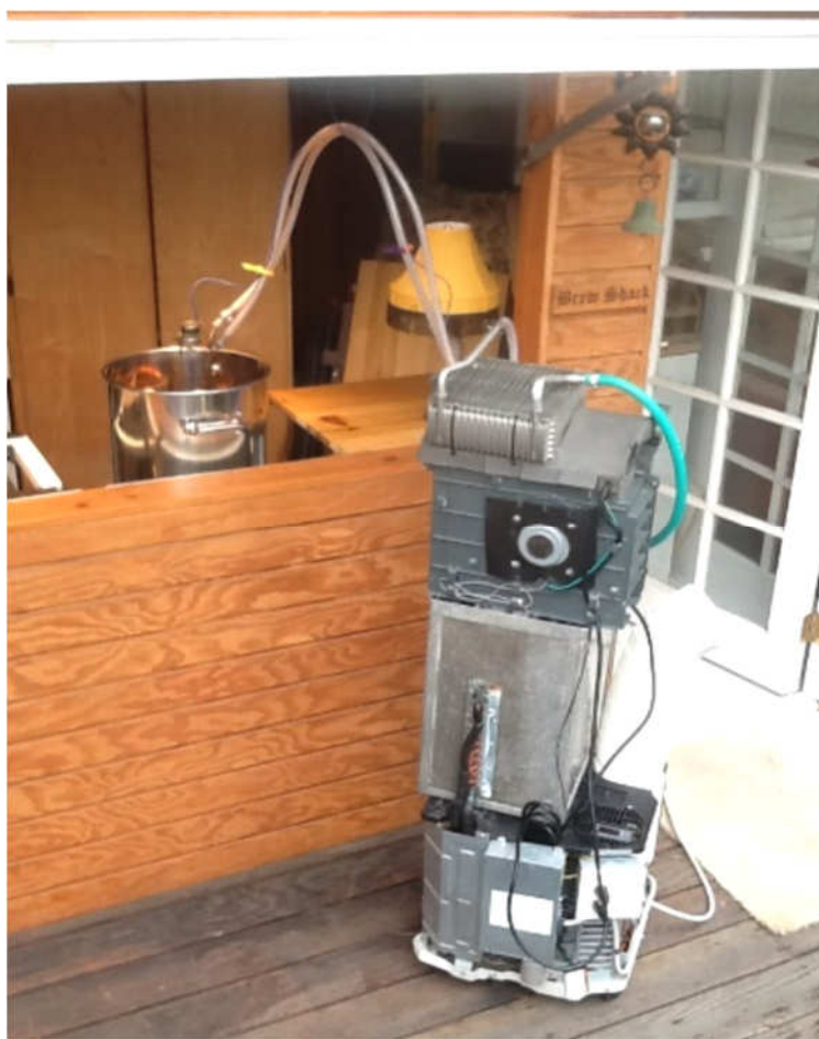
The Frankenchiller - Don't be scared, it saves water- really
