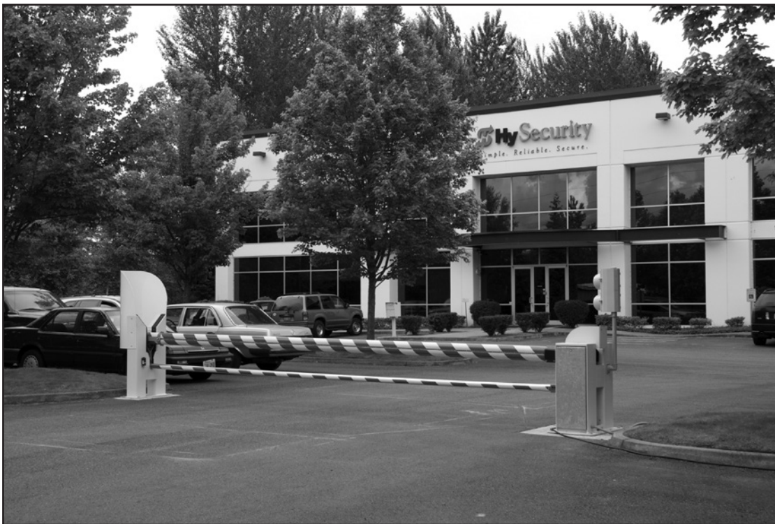
HySecurity Gate, Inc. Headquarters in Kent, WA
