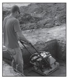
Soil Density compacted to 95% per ASTM-698
