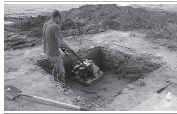
Soil Density compacted to 95% per ASTM-698
