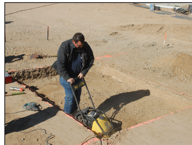
Compact soil and prep drainage channels
