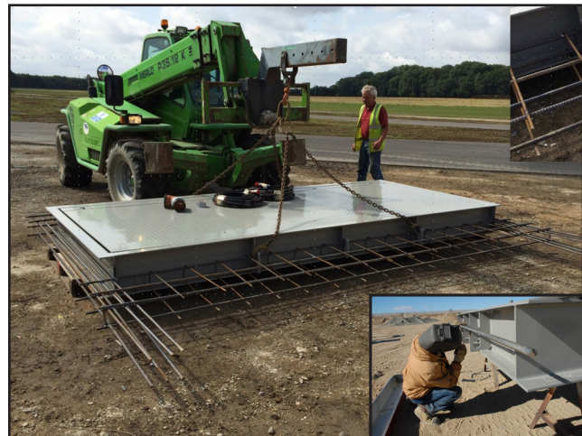
Transport base and assemble rebar reinforcement
