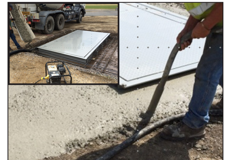
Remove air pockets. Smooth and finish.
