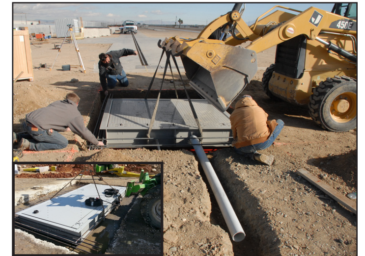
Place HydraWedge SM50 in foundation pit
