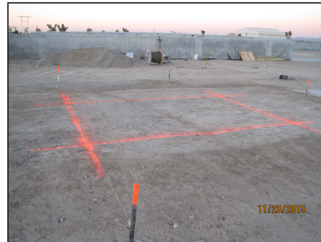
Designate site layout for resurfacing
