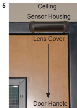
Install R2E-100 with Lens Cover Facing Down Toward Door Handle
