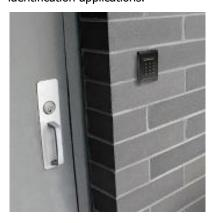
**Features** The keypad's output is field-programmable for either 4- or 8-bit key bursts or 26-bit code transmission. The reader's 2-color LED and beeper are controlled by the reader itself. No external wiring is required for this feedback.
