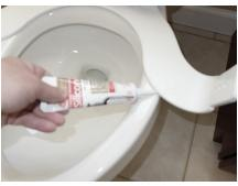
Place a bead of silicon caulk around the outer edge of the Comfort Arms base plate in the front and the back. This seals the base plate for easier cleaning.
