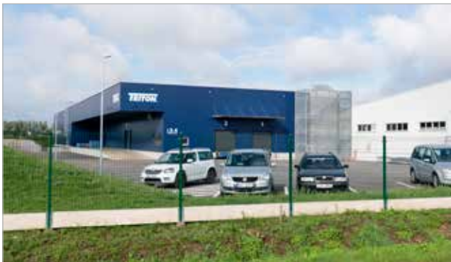
On January 2022, a new production hall with a usable area of nearly 3,000 m 2 was approved.
