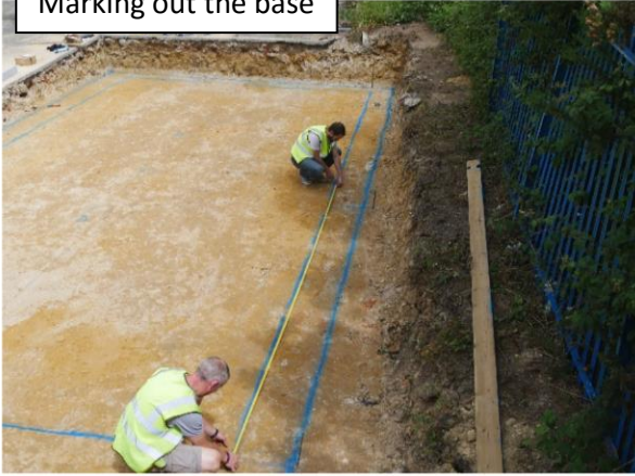
Marking out the base
