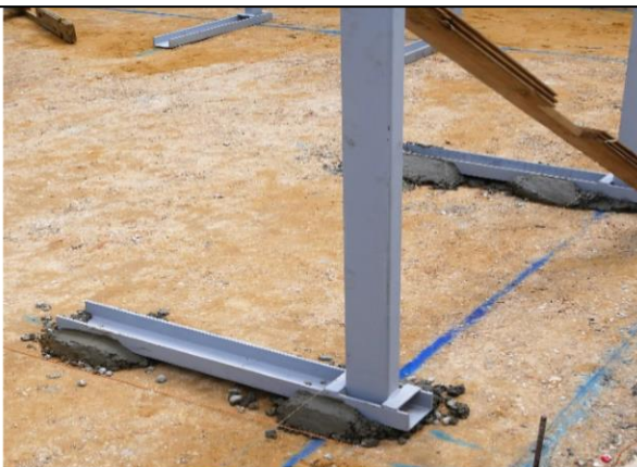
A brace secured in position with a bed of mortar.
