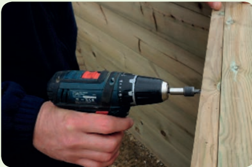
Fitting the Shelving Support
