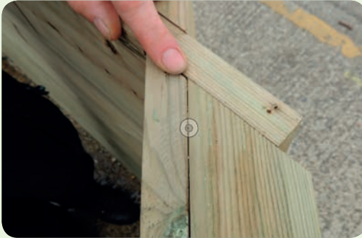
Top view of Shelving Support in place
