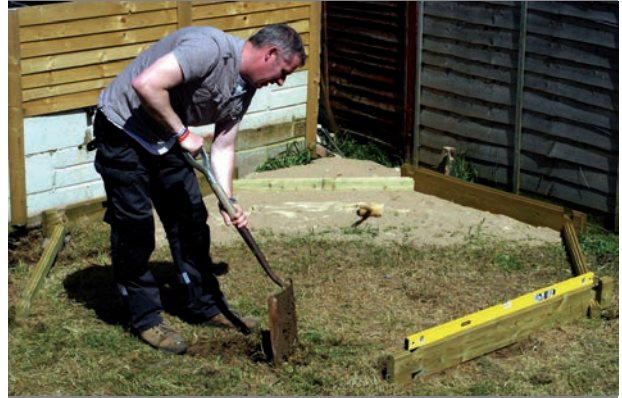
Prepare the ground
