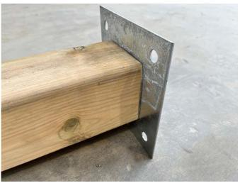
Four screws into bottom of plate
