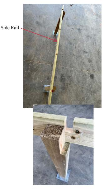
• The side rail with multiple notches joins onto the side of the post with the deepest notch. Lay posts approx. 3m apart and fix a side rail onto the deepest notch with the end groove of the rail in line with the higher groove. This is so when you start inserting the runners the end ones sit tight against the post. Once positioned use the small 6mm drill to pilot hole the rail and use 2no 3" screws to fix in place
