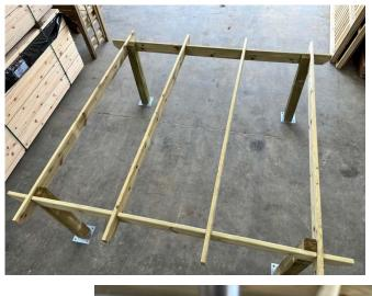
• Now place opposite the other two posts and rail and start inserting the runners and fix in place by drilling a pilot hole then use the 3" silver screws to hold in place.
