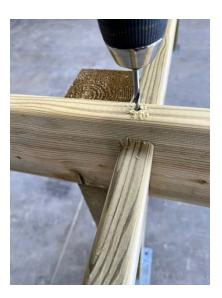
• There are two wood diagonals to go at each corner. Predrill approx. 1" from each end and fix in place using 1no gold screw. They also help square up the posts and keep the pergola/lean to more stable.
