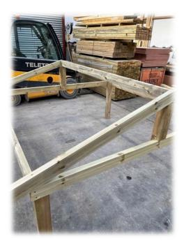
8. To fit the trusses always start from the top on both sides. You will see we have already marked the positions on the outer and centre frames. Pre drill the frame and fix with just 1no 100mm screw as this is all that is required, the second one will go next to this one and will need to be screwed in at an angle due to the opposite one being in the way.
