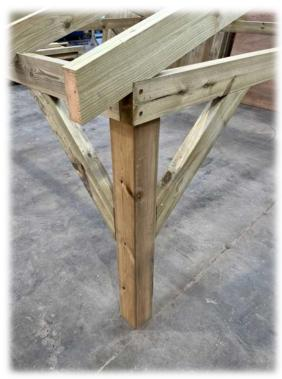
12. Your framing kit is level and fixed in position. You now need to fit your 2-side fascia's. Pre drill and fix in place with a 3" screw at the end of each truss.
