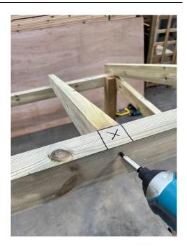
8. Once the centre trusses are in place you can now screw them to the outer frame. If the frames are bowed or twisted either pop the framing into the notch or pull the framing to the outside so it's as flush as can be. Pre drill through the top of the truss and fix in place with a 150mm gold screw.
