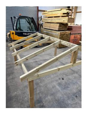
10. Make sure your posts are level and fit the corner braces. Pre drill at each end and fit in place with the 100mm gold screws.
