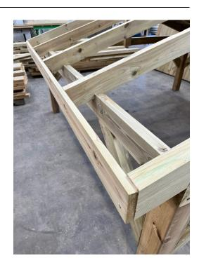
12. Starting from the bottom overhang the first Featheredge board 25mm and fit in place with stainless steel nails. We recommend 2 nails at each truss. Place the next board on top so that there is a 30mm overlap and repeat the nailing process. Repeat this until you reach the top. Repeat on the other side. How you finish the overlap at the top is your choice but we believe to overlap the two top most boards is favourite.
