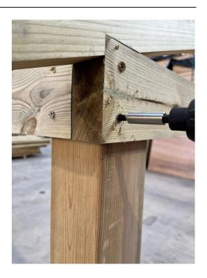
6. Insert the centre rail which has two pre-positioned L brackets attached. Place centrally on the post and fix in place with 4no 40mm screws at both ends
