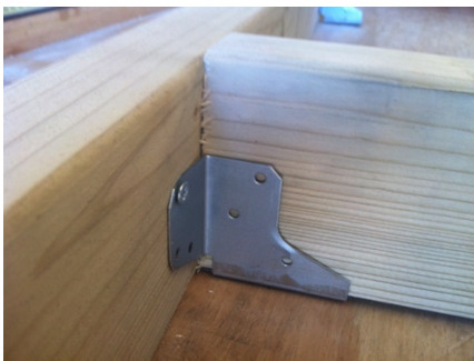
Joist hanger view
