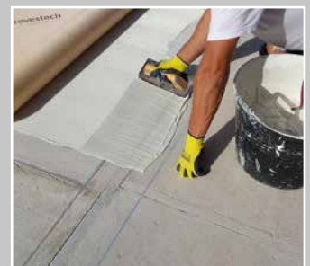
Waterproofing of terraces with DRY80 . MELIÁ GORRIONES FUERTEVENTURA****. Fuerteventura (Las Palmas_ Canary Islands).
