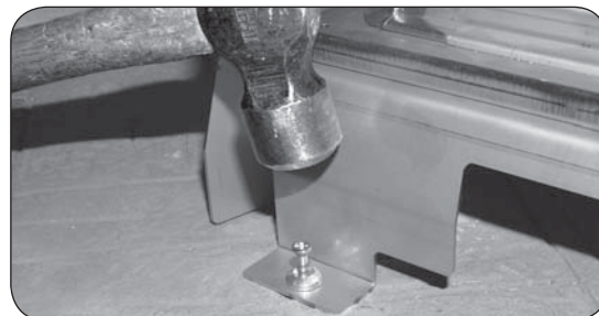
Fig. 16-3 Install hammer screws
