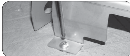
Fig. 16-2 Fasten hammer screws
