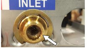
**3.** Remove the cover. Connect the pre-assembled inlet and outlet pipes to the heater and fully open the inlet and outlet ball valves. Check for water leaks. If a leak is at a compression fitting, slowly tighten the compression nut until it stops. Replace the cover.
