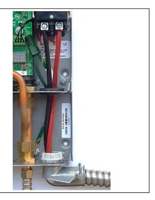
**2.** The power leads are to be secured to the L1 and L2 or L and N connectors on the terminal block or relay. The ground lead is to be secured to the GND connector on the block or the green ground wire with the provided wire nut.
