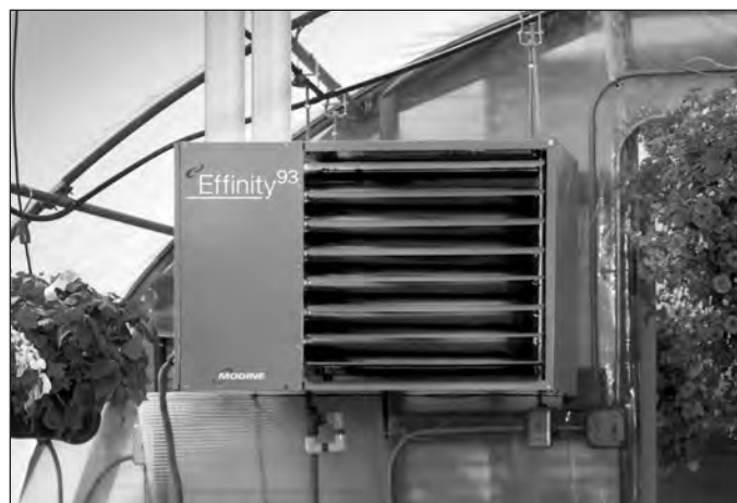
At 93% thermal efficiency, the Modine Effinity 93 is North America's most efficient and complete unit heater line and an ideal solution for offering greenhouse operators substantial savings on their fuel costs.
