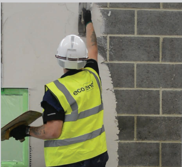
Apply with trowel to blockwork wall
