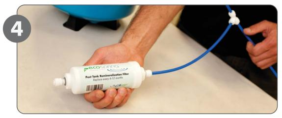
4) Insert tubing to 1/4" tee, then insert tubing into remineralizing post filter.
