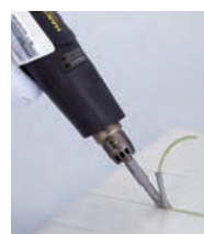
Welding floor coverings Use of nozzle holder and V type nozzle
