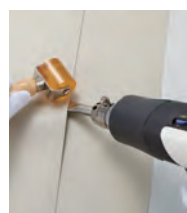
Welding PVC sheet Use of nozzle holder and spatula type nozzle along with roller
