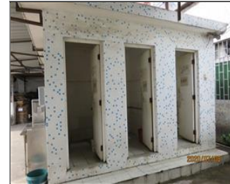
Photo of the sanitary facilities toilets.JPG
