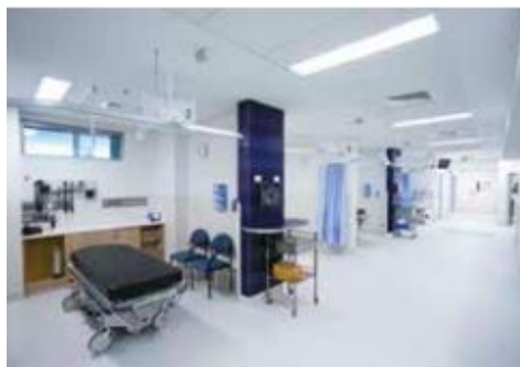
Geelong Hospital - Vinyl installed at the Geelong Hospital Emergency Department after the concrete was levelled with Ultraplan
