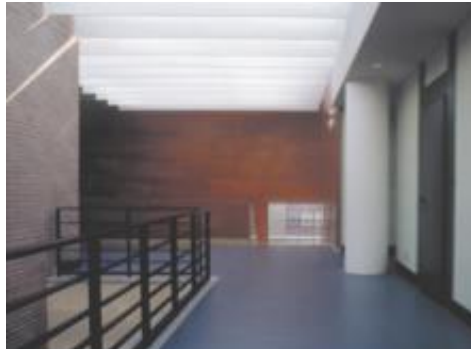
An example of an installation of linoleum on a surface levelled with Ultraplan - Monzòn Conservatory - Spain
