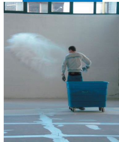
Throwing Quartz 0.9 AU into wet Mapeproof 1K Turbo
