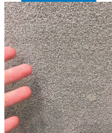
All loose sand removed and final surface completely saturated
