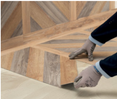
Installation of MODULAR LVT with Ultrabond Eco V4 Evolution
