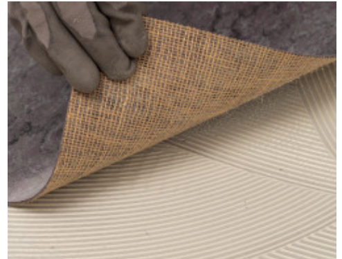
Installation of Linoleum with Ultrabond Eco V4 Evolution
