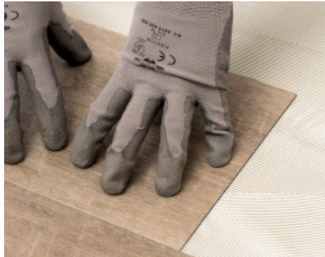
Installation of LVT with Ultrabond Eco V4 Evolution
