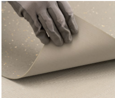
Installation of RUBBER with Ultrabond Eco V4 Evolution
