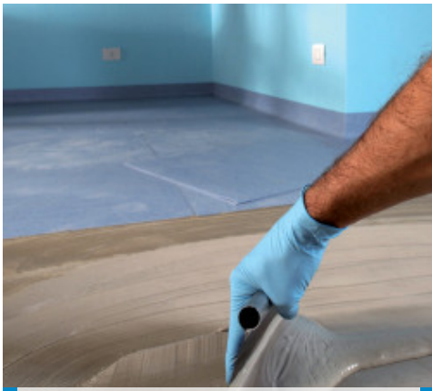
Applying Ultrabond Eco 380
