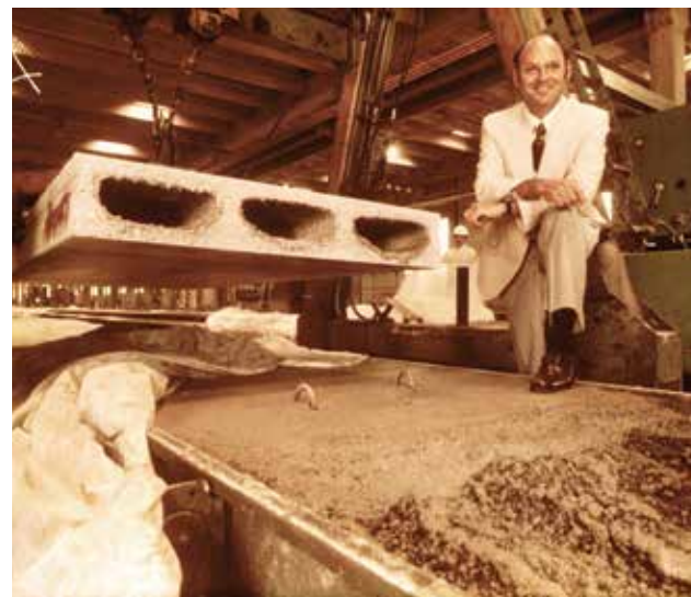
William K. Nitterhouse is photographed here for an ad in Life Magazine for an insurance company. He is standing beside a hollow core plank – one of the main products that we still produce today.
