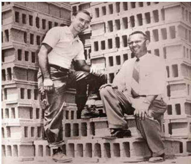
T.K. Nitterhouse, 2nd generation (seated) and William K. Nitterhouse, 3rd generation. This photograph was taken for an article in a local newspaper. William K. Nitterhouse began running one of the block plants at age 19 and continued to build the company into what it is today.
