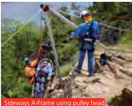
Sideways A-Frame using pulley head
