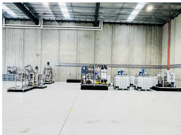
Figure 1d: Large-scale pilot plant equipment being assembled.
