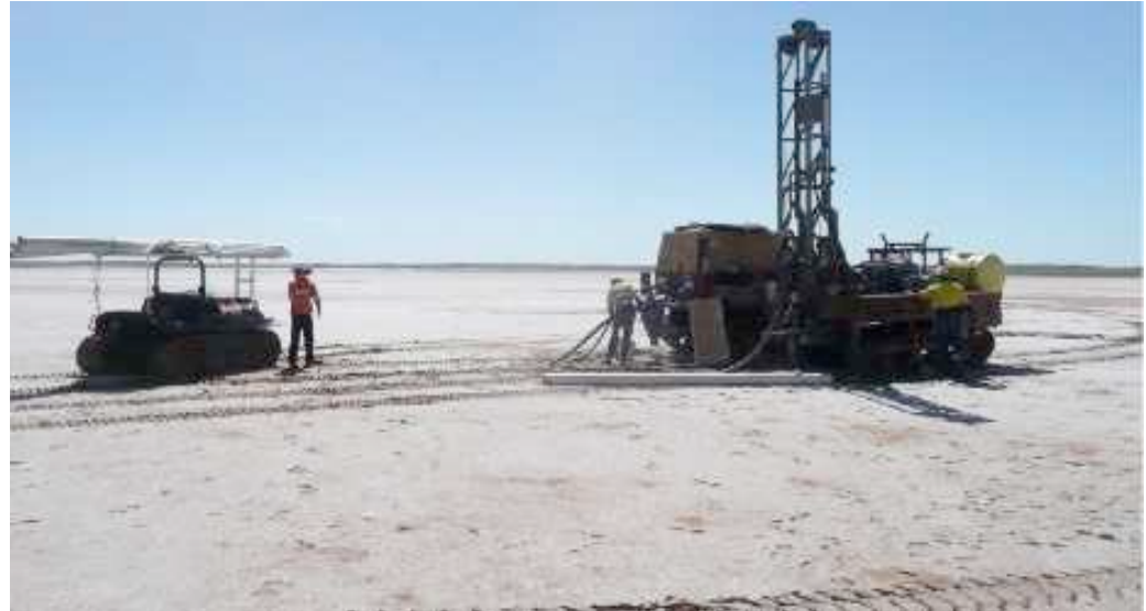
KLPP Project Evaluation - extensive drilling, sampling & investigative studies
