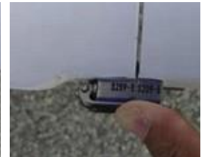
Fold down latch to top surface and secure it so that petals are connected to each other.
