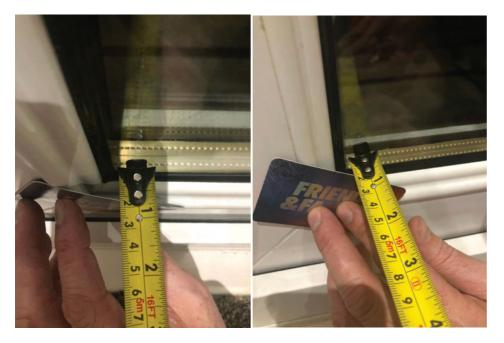
4. Lastly, measure the depth of the window from glass to beading. To do this, simply place a credit card over the corner of the frame and use a metal tape to take the measurement. This size can range from 18mm up to 38mm.
