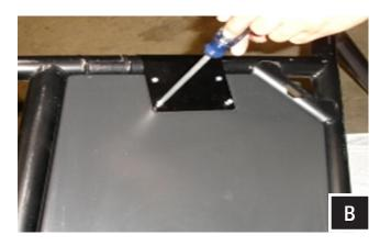
B. While holding the enclosure securely in place, loosely install the 2 brackets using the screws provided.
