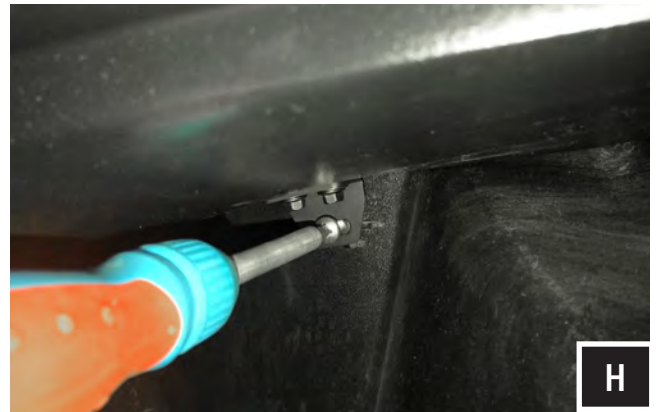
H. Fasten the provided #14 screw to secure the enclosure lower mounting bracket.
