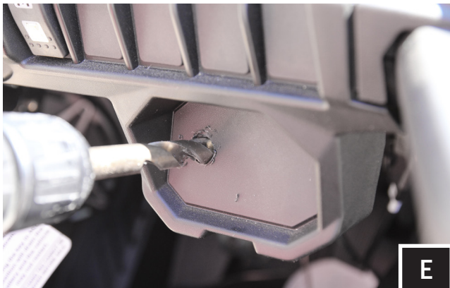
E. Using 9/16" drill bit, drill hole off set to the left of the dash for the MRB3 controller cable.
