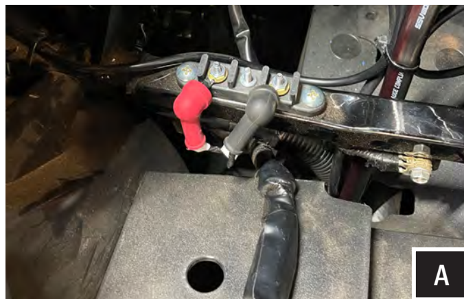
A. Run power and ground to busbar.
