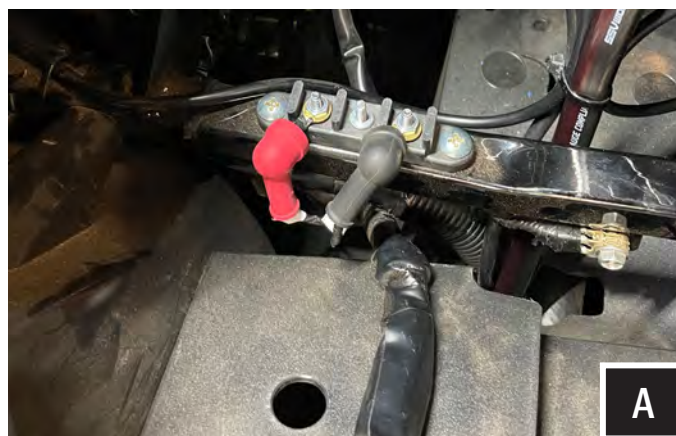
A. Run power and ground to busbar.
