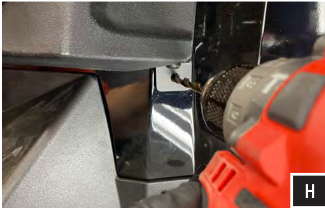
H. Using the guide left by the punch tool, drill a hole using a 1/4" drill bit
