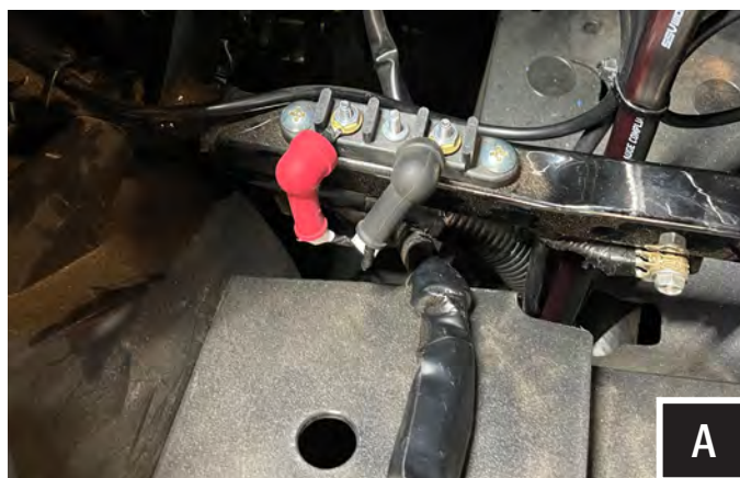
A. Run power and ground to busbar.
