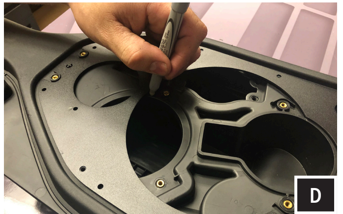
D. Set the adapter base plate onto the disassembled sound bar. With a permanent marker or paint pen, outline the perimeter of the adapter base plate to create a cut line.
