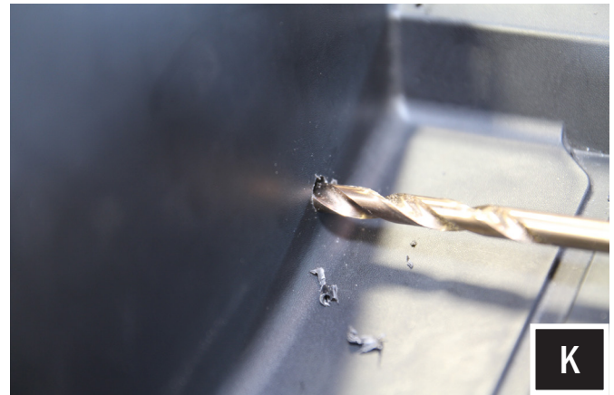
K. Follow through the pilot hole with a 5/16" drill bit.
