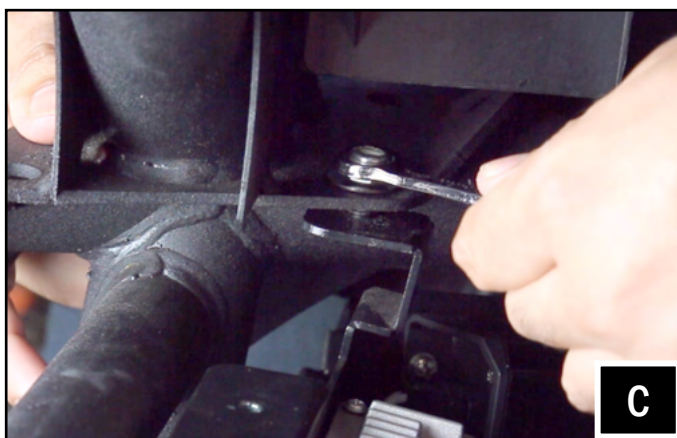
C. Secure the amp tray to the vehicle's ROPS cage using the supplied M6 flange hex head Bolt, 10mm nut and washer.
