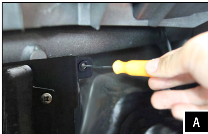
A. Make a pilot hole with a pick tool through the top right screw hole in the amp plate and push all the way through the vehicle panel.
