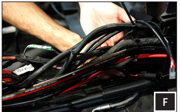
F. Run the rear speaker and subwoofer cables along the passenger side of the center console. Use zip ties to tidy up the install.
